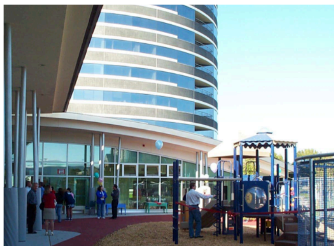
South San Francisco built a child care center in an office park to support the growth of its biotechnology industry.
