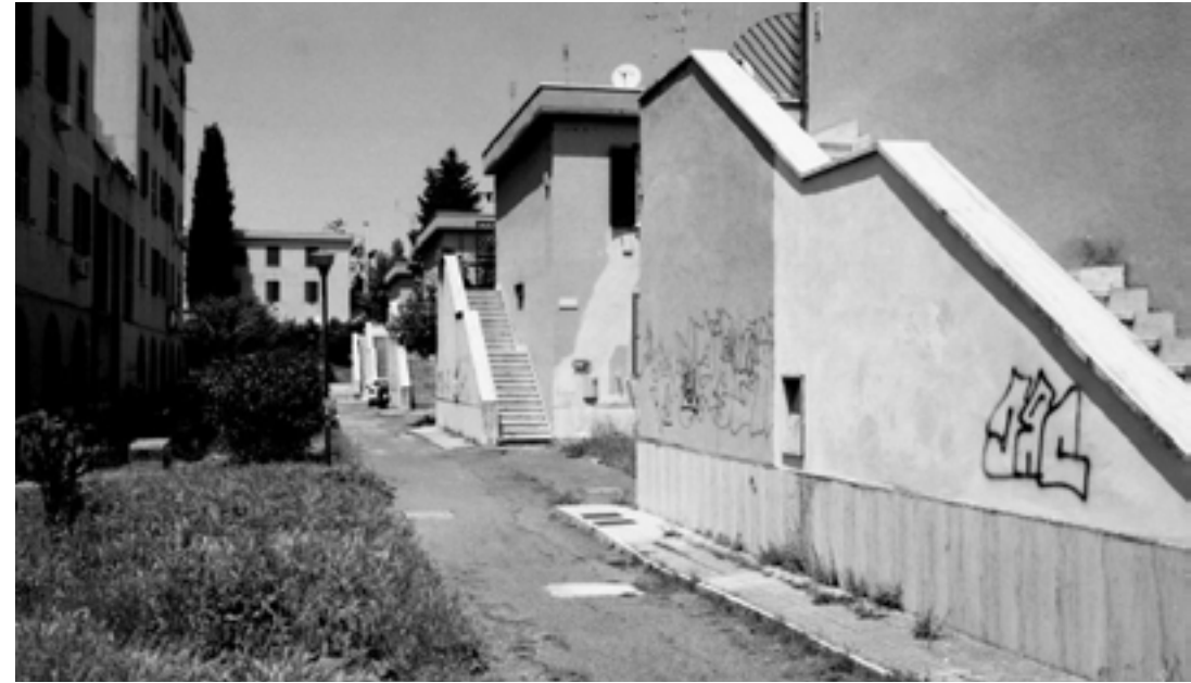
This modern photograph shows the two-floor flats characteristic of the western end of Tufello's older housing core, the 'trapezoid'. Apartments occupy only a single floor and so the staircases and the public balconies they lead to are the only entrances to the upper floor apartments. Photograph by Simona Mizzoni.
