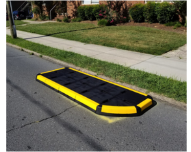
Temporary curb extensions
