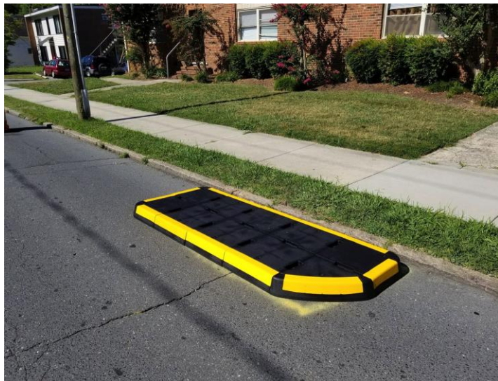
Figure 3: A plastic and rubber temporary platform installed as a curb extension in Bethel, Vermont. Source: Better Block Initiative.
