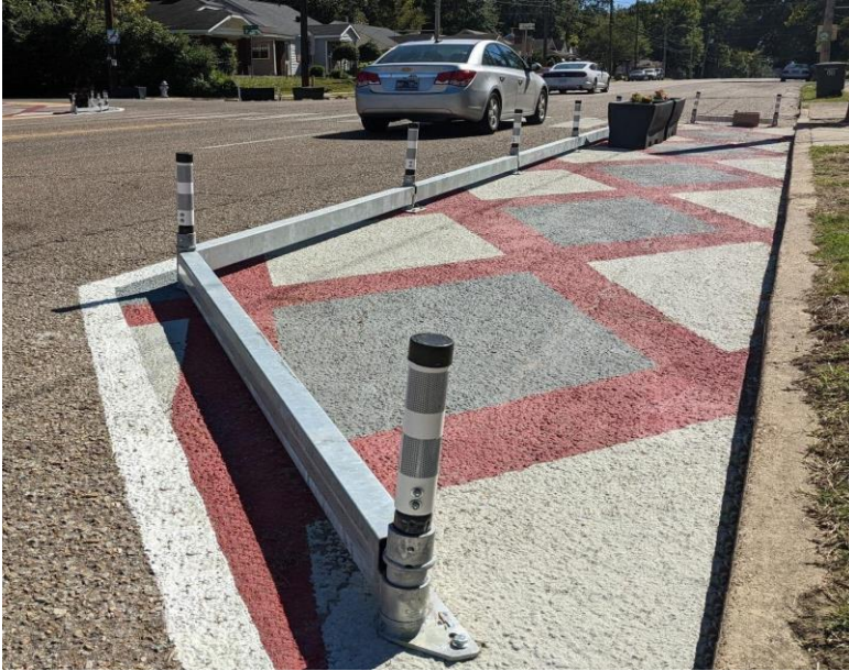
Figure 2. A temporary curb extension composed of painted pavement protected by metal posts in Nashville, Tennessee. Source: Complete Streets USA.
