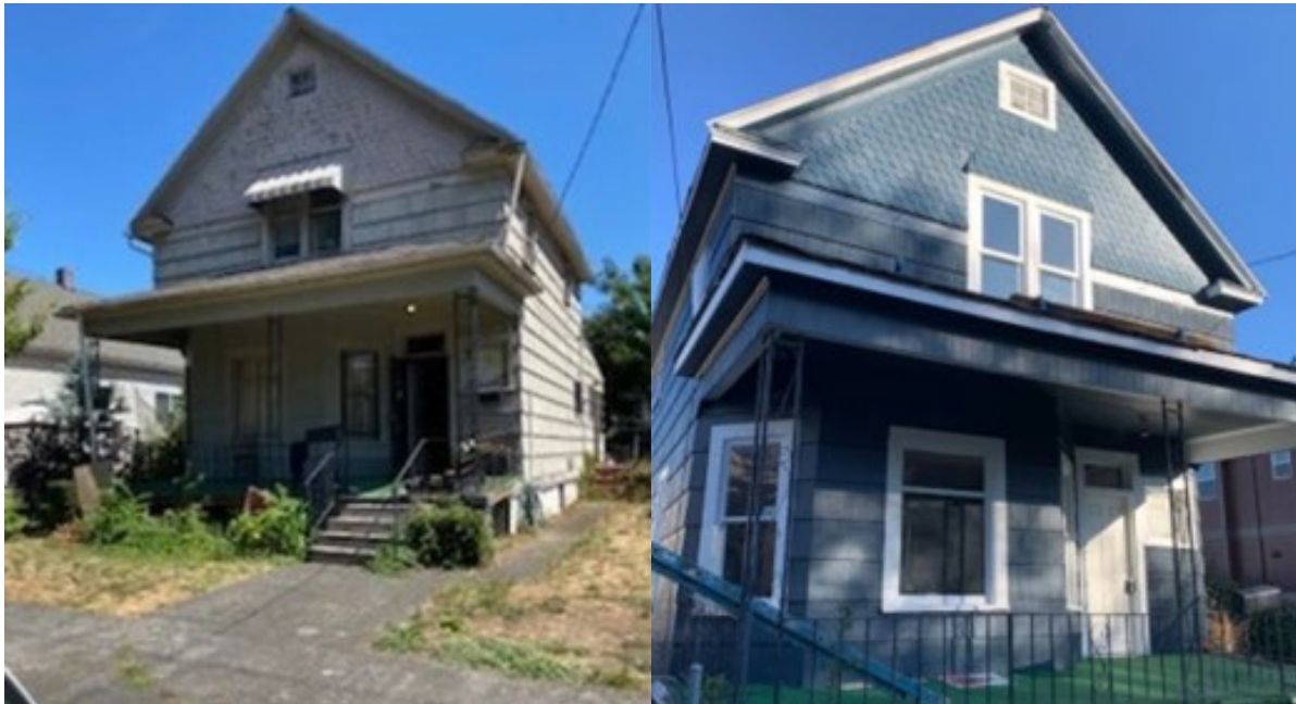
Image 4. BIPOC community members and those with disabilities receiving code violations in Portland, OR, can seek free assistance from the City. Pictured here is a before-and-after photo of a property. City of Portland
